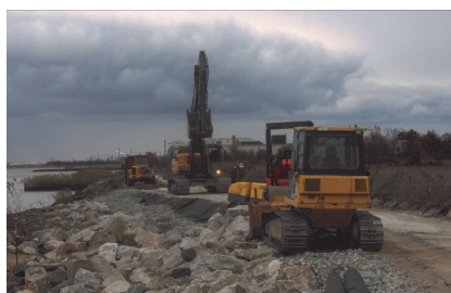
Rock being installed by K. C. Construction on the Army Creek Dike project south of New Castle in November 2013.
