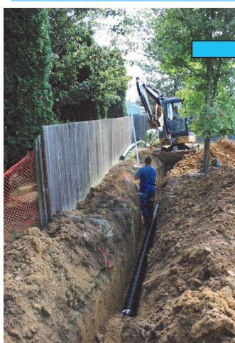
Drainage system being installed in Huntington subdivision near Newark
