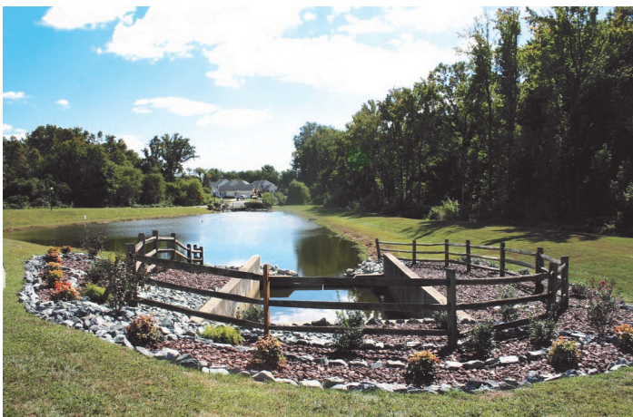
An eroding area at this stormwater pond in The Estates at Red Lion was protected with landscape stone and riprap.
