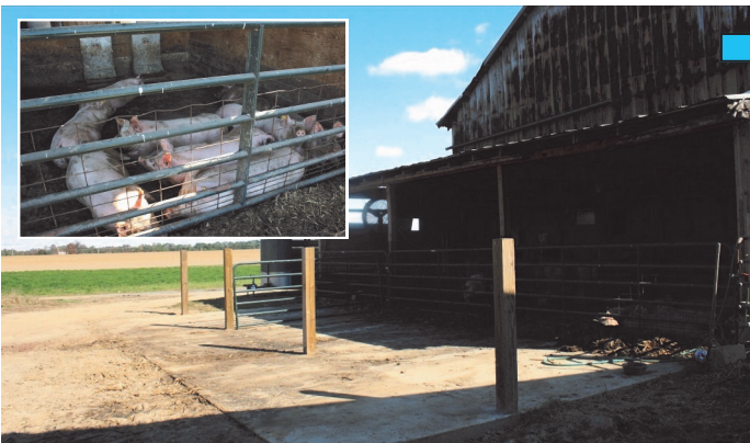
This heavy use area concrete pad provides a place for the farmer to clean up the animal manure from his herd of pigs.
