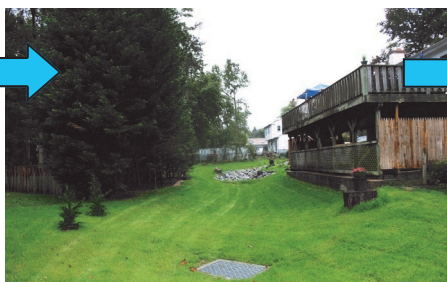
The area was then seeded and stabilized using erosion control mat
