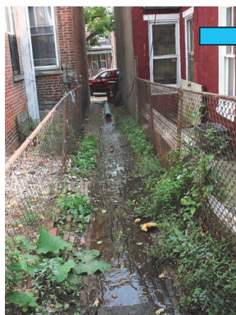
Constantly running water down this alleyway caused icing on West 5th Street in Wilmington
