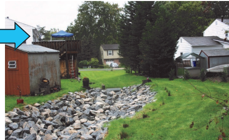
The upper section of the drainage ditch was protected with riprap
