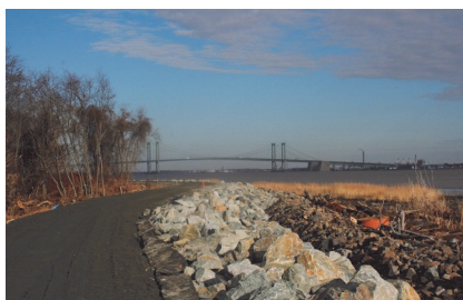
Riprap protection along a section of Buttonwood Dike looking towards the Delaware Memorial Bridge. Work by Merit Construction Engineers.
