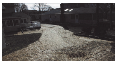
Swale and enclosed drainage system in the Four Seasons community near Newark
