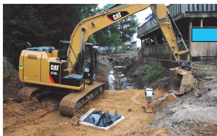
An eroding drainage ditch behind this home in Piermont Woods near Newark is being piped with a lawn basin
